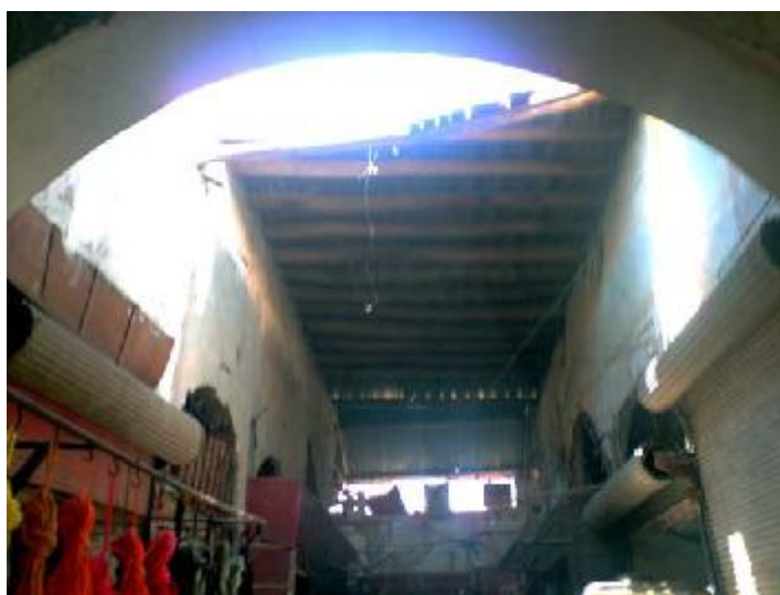
Left, crack showing the separation of the back wall from the cross wall in a shop in the souk.
