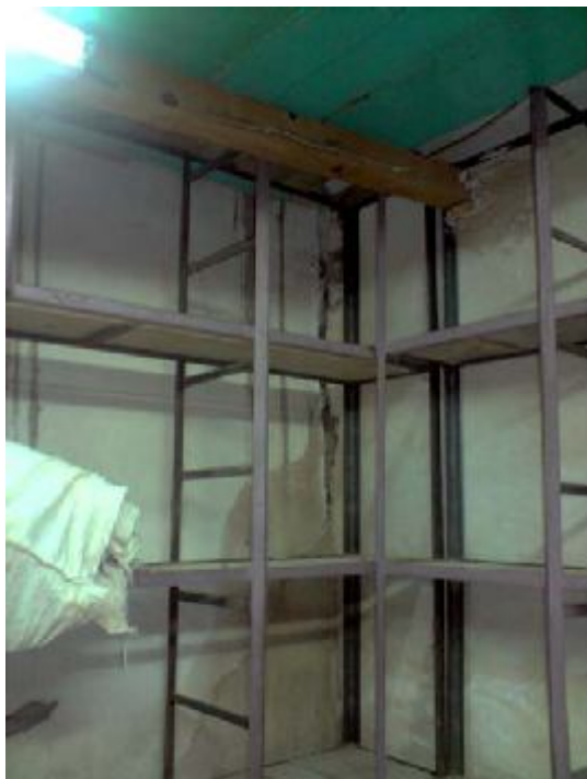
Left, crack showing the separation of the back wall from the cross wall in a shop in the souk.
