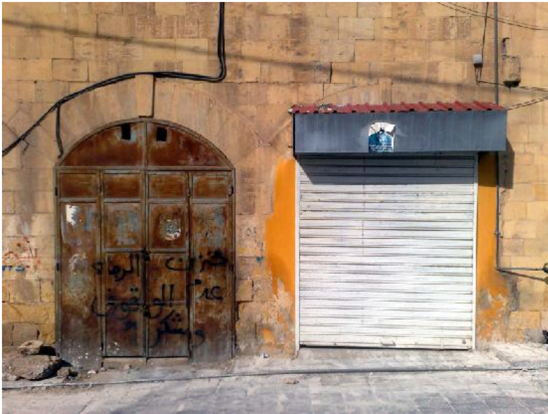
Above , pair of historic shops in Salt, Jordan. On the left, historic iron shutters leave the architecture visible, while in the case of the shop on the right, the modern face-fixed roller shutter completely conceals the arched shop front. In this case, the leaves of the iron shutters are wider than those identified elsewhere and recommended for use in Deir Ezzor.
