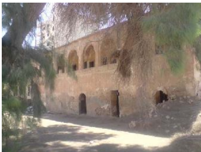
Above right, northern, rear, elevation of the Saray gateway, showing the collapsed vaults.
