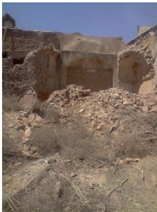
Above right, northern, rear, elevation of the Saray gateway, showing the collapsed vaults.
